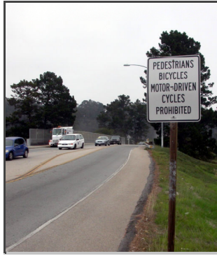
Approaching the Morrissey bridge from the South
